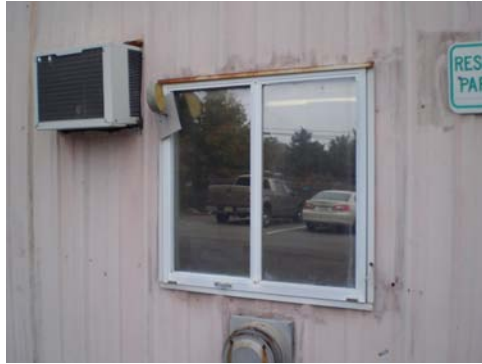
Damaged/ aged window frame and air-leakage at sleeved wall air-conditioning units
