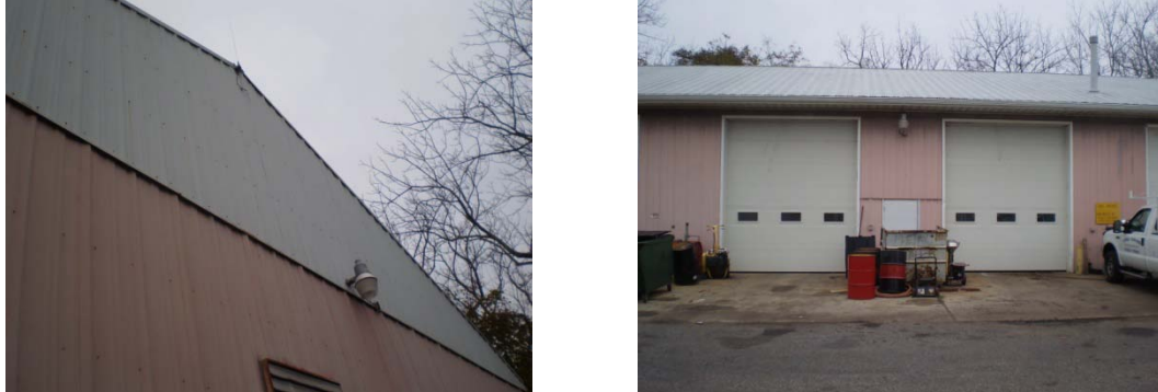
Typically found aluminum exterior walls
