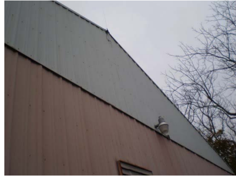
Partial South Façade
