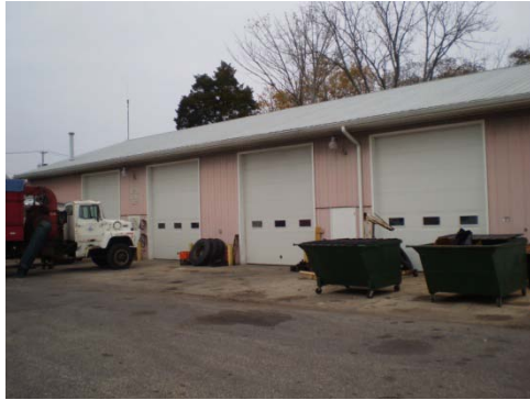
Partial West Façade
