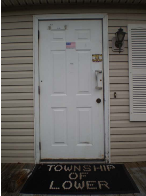
Partially missing/ worn weather stripping
