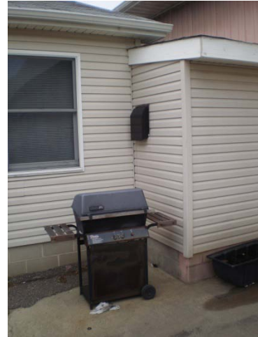
Partial North Façade
