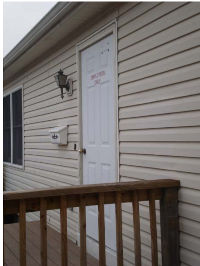
Partial East Façade
