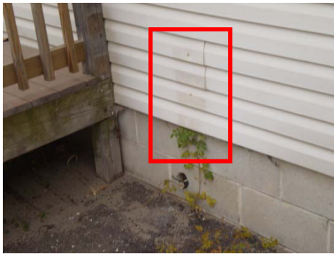
Signs of water damage at perimeter walls and damaged metal siding
