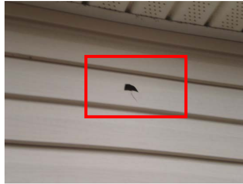
Signs of water damage at perimeter walls and damaged metal siding
