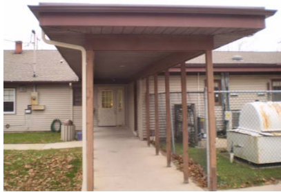
Partial West Façade
