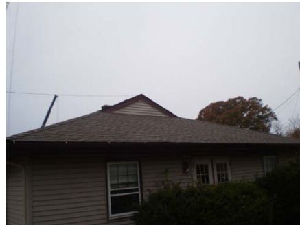
Partial North Façade
