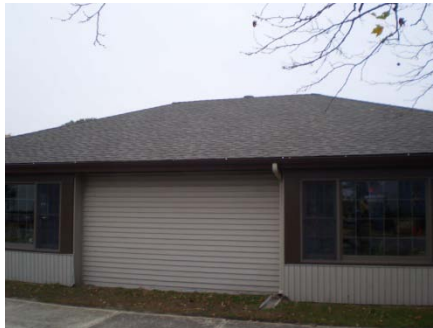
Partial South Façade
