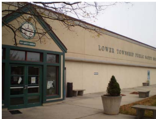
Partial South Façade
