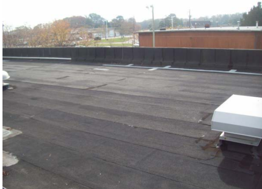
Built-up bituminous finish
