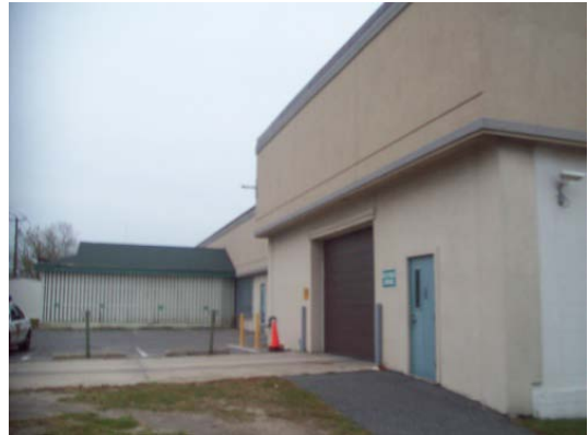
Partial East Façade
