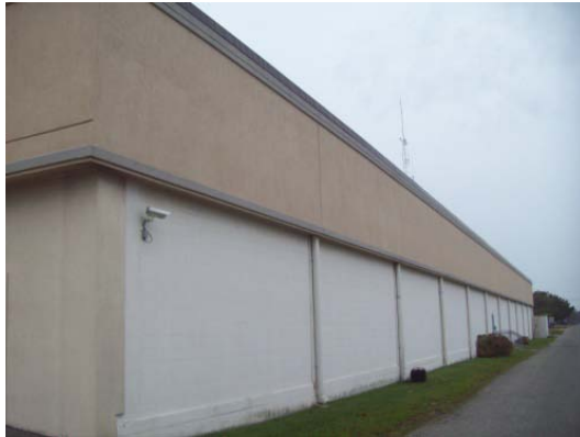
Partial North Façade
