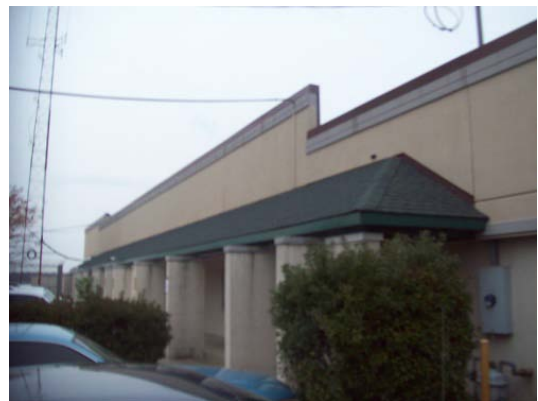
Partial West Façade
