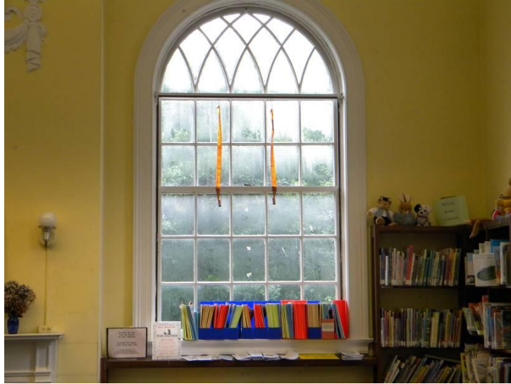
Original Building Existing Windows
