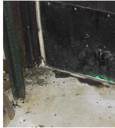
Missing or Worn Weather-Stripping at all Doors
