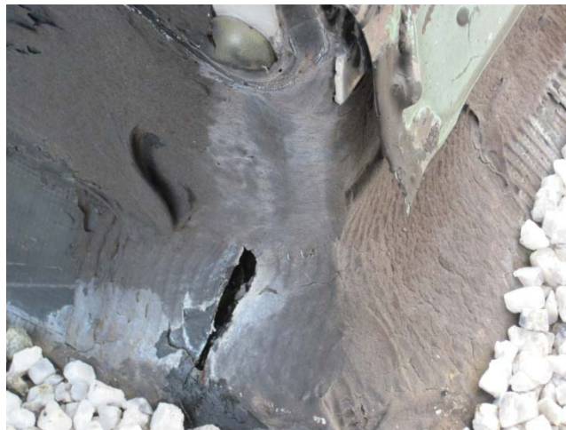
Cracked membrane at roof corner
