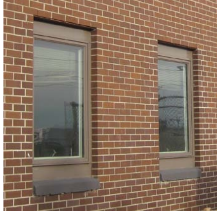
Double Aluminum Window panel wall system
