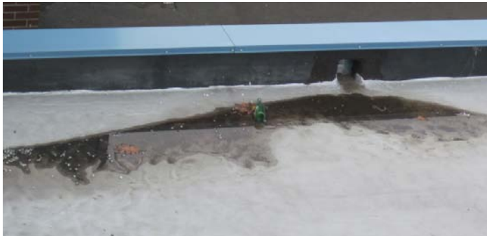
Pooling on roof and area of built-up missing gravel
