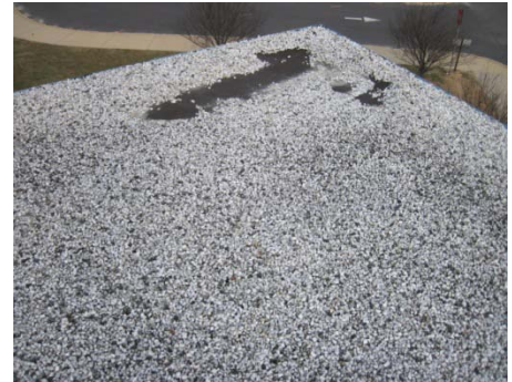
Pooling on roof and area of built-up missing gravel
