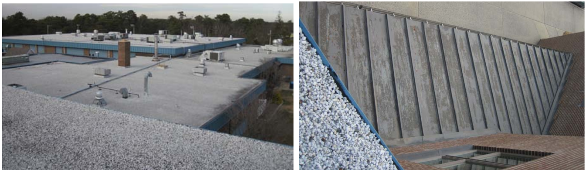
Built-up roof at OCVTS; Metal seamed roof above side entrance
