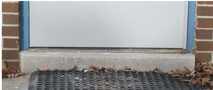
Verify seal at threshold of door
