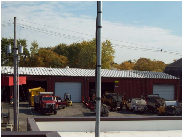
Existing Roof above the Garage
