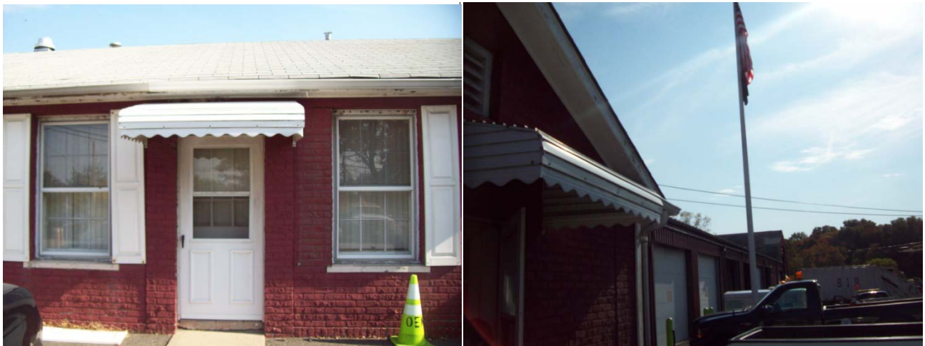
Existing Exterior Walls
