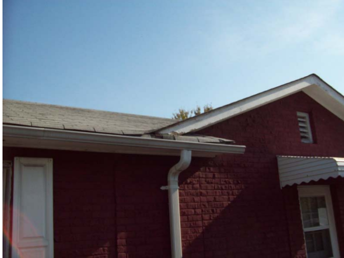
Existing Roof above the Office Building
