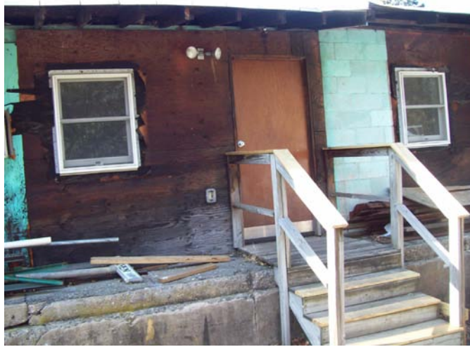
Rear Wall under Construction
