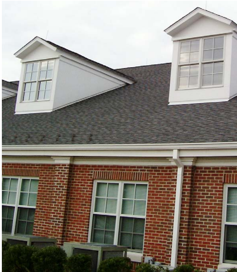
Example of typical installed windows
