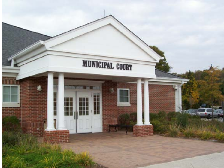
Existing Exterior Walls
