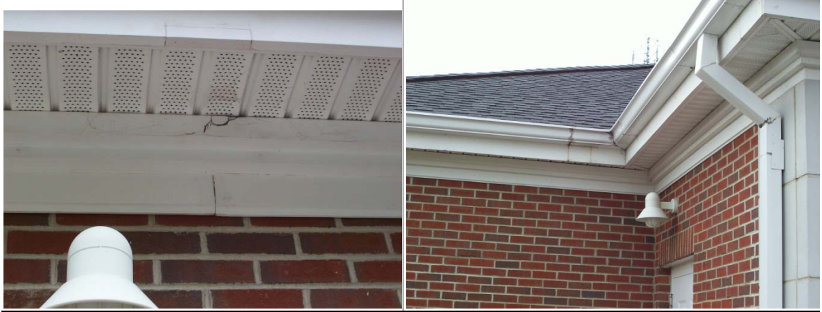
Example of damaged roofing eave
