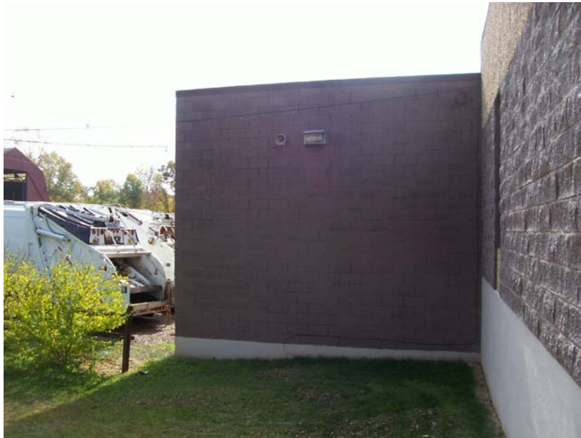
Existing Exterior Walls
