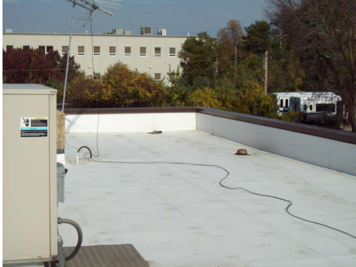
Existing Built-up Roof
