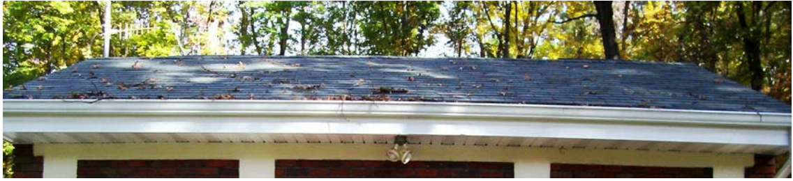
Existing Roof Surface
