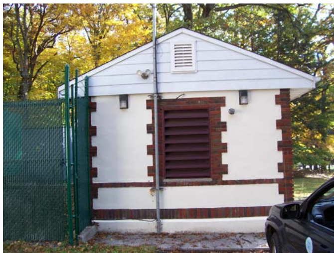
Existing Exterior Walls
