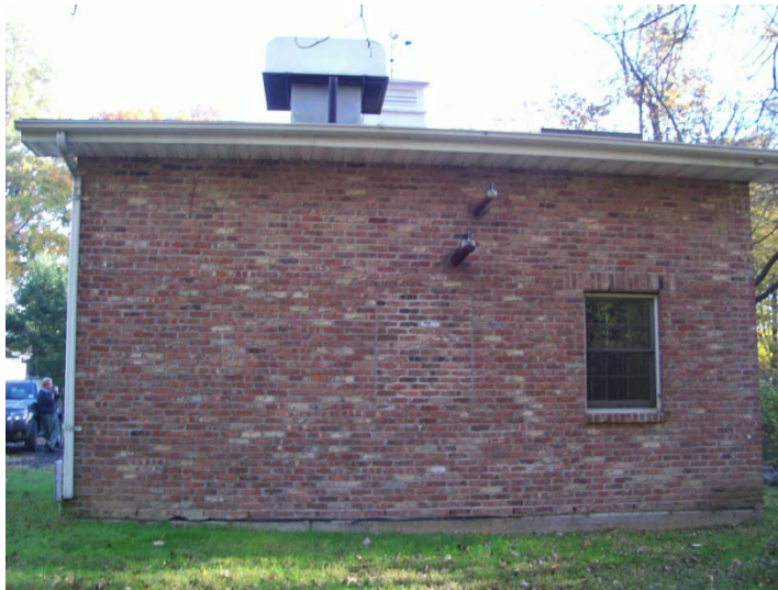
Existing Exterior Walls
