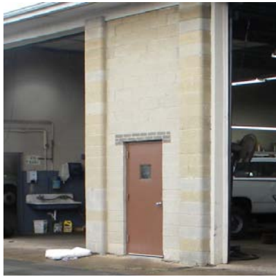
Image of garage bays and metal door.
