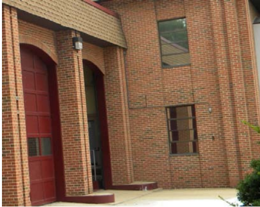
Typical existing windows
