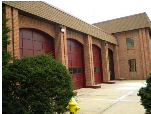
Typical exterior surface at the firehouse
