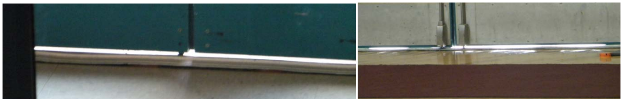
Doors showing need for higher threshold, door sweep or weather-stripping – main door and gym doors
