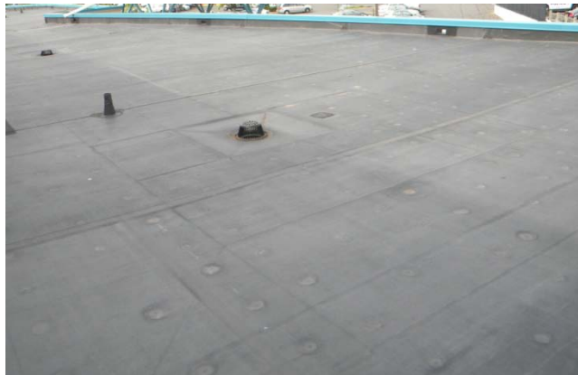
Image of roof membrane in age appropriate condition
