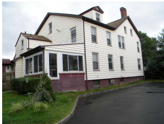
Typical exterior wall surfaces
