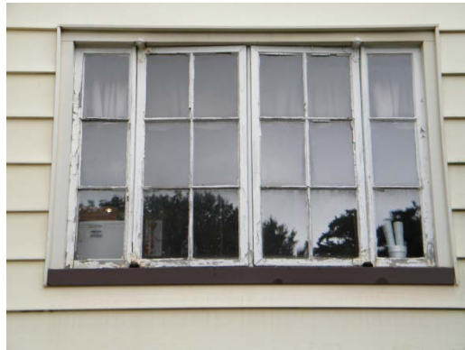
Typical original windows
