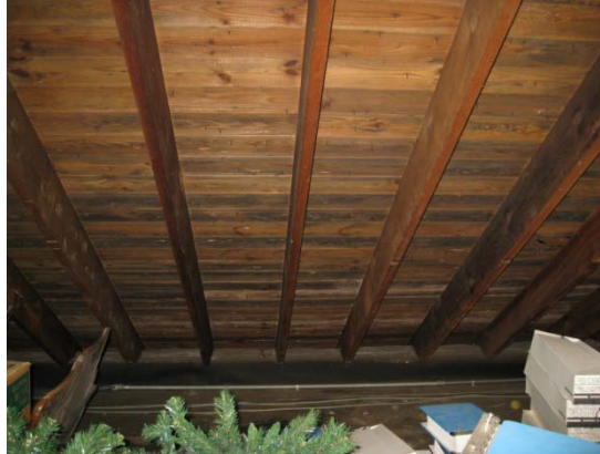
Wooden trusses that form roofline
