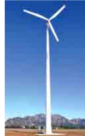
FINAL - Energy Audit Report, May 2010
