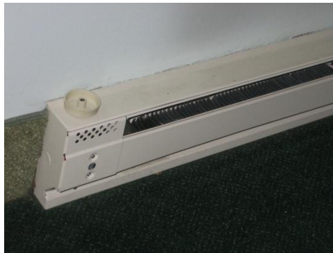
Typical Baseboard heater
