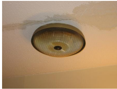
Typical bathroom heating
