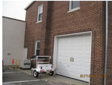
Partial Rear Façade (typ.)
