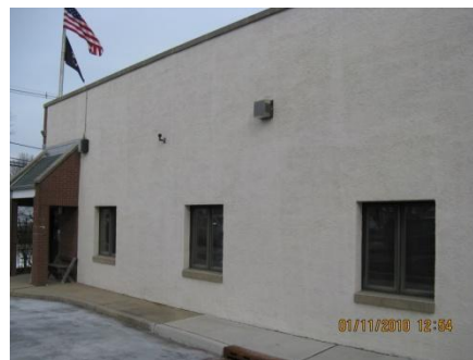
Partial Right Side Façade (typ.)
