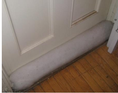
Damaged / warped / aged door frame
