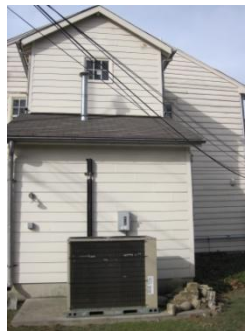
Partial Rear Façade
