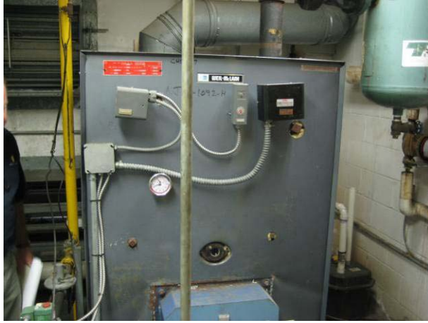
This boiler provides heat Electromechanical thermostat
