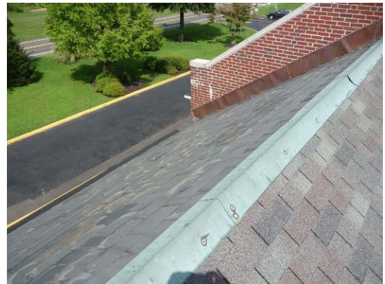
Aged Slate Roof on left
