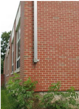
Missing downspouts and areas of brick veneer damage due to water/ moisture infiltration
