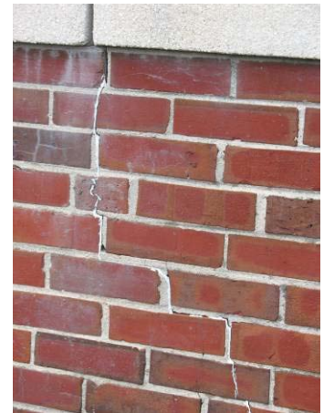
Missing downspouts and areas of brick veneer damage due to water/ moisture infiltration
