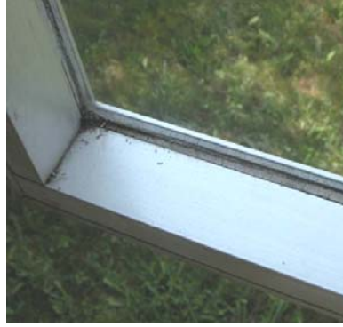
Original single glazed aluminum framed windows
