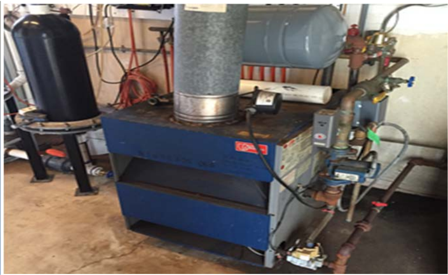
Indoor Pool Utica Cast iron Boiler
