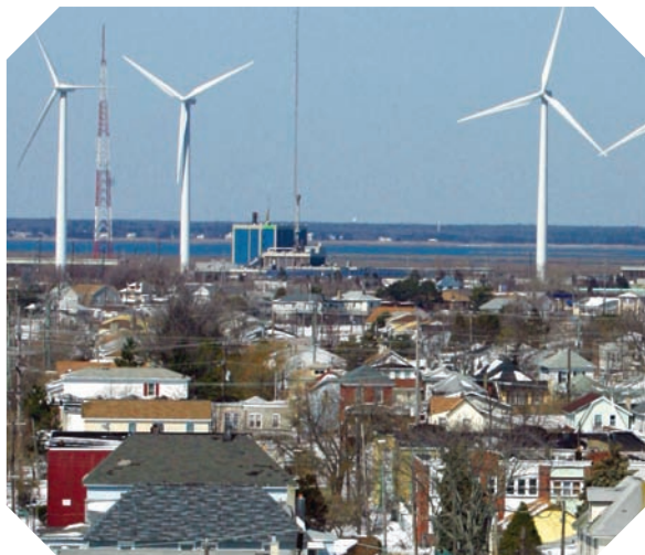
The Atlantic County Utilities Authority's wind energy project includes five 1.5 MW turbines visible from the Atlantic City Expressway.
