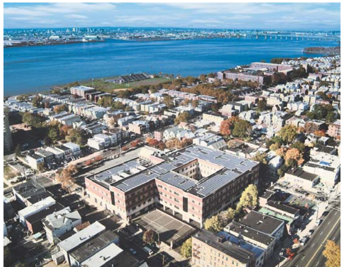
Aerial photo of Bayonne High School: Almost 10,000 solar panels will be installed on nine Bayonne schools.
