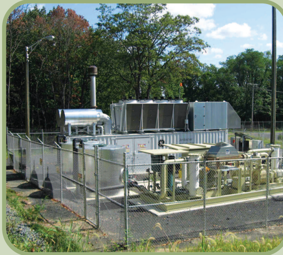
Monmouth County's one megawatt sustainable biopower project produces enough energy to support their materials processing and recovering facility.
