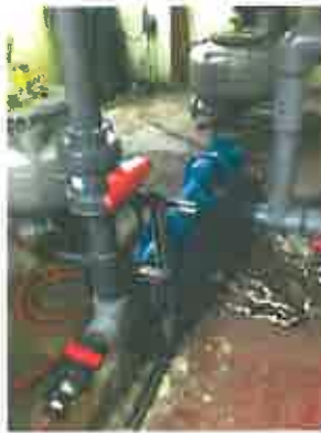
(c) Monyo Progressive Cavity Pump
