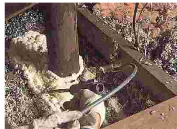
Sealing Air Leaks around Plumbing Chases
