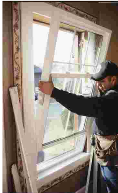
Low-E Windows help keep heat inside during winter, outside in the summer *
