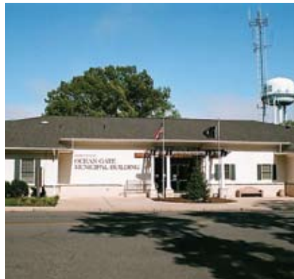
Borough of Ocean Gate's Municipal Building
