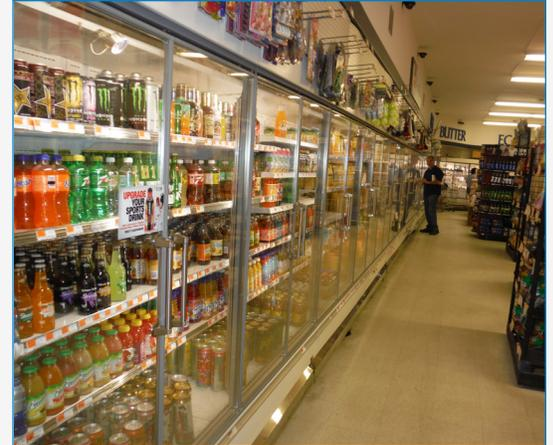
*Doors on dairy cases and night curtains on meat and produce cases as well as new refrigeration controls, motors and LED case lighting at the Farmingdale Shop n Bag resulted in an estimated 30 percent reduction in energy use.*
