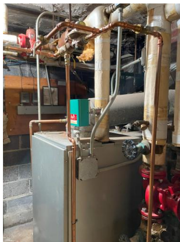
Boiler and Uninsulated Piping
