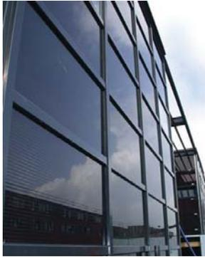
EPV Solar offers aesthetically appealing PV modules, which can easily be integrated and replace standard architectural materials for cost benefits.
