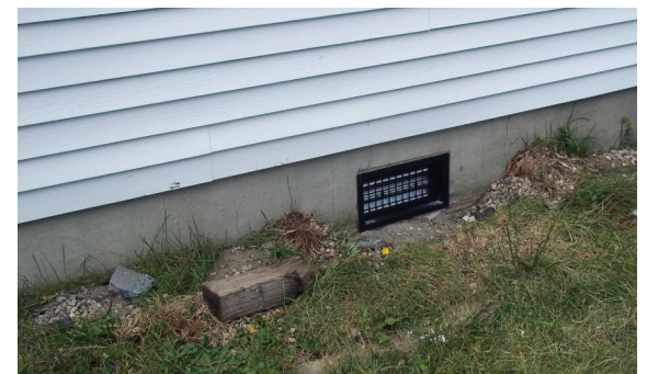
New crawl space vents around the foundation provide better ventilation and help to eliminate moisture issues.
