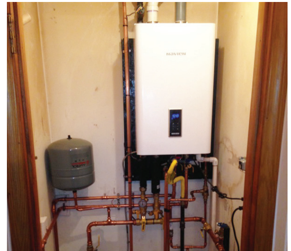
The new wall-mounted heating system combines boiler and water heater in one energy-efficient, space-saving unit with easy controls and increased comfort.
