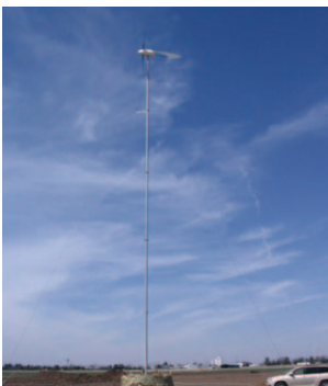
Guyed Monopole Tower
