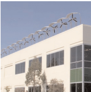
AeroVironment rooftop array
