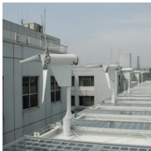
Proven Energy 2.5kW turbine rooftop array
