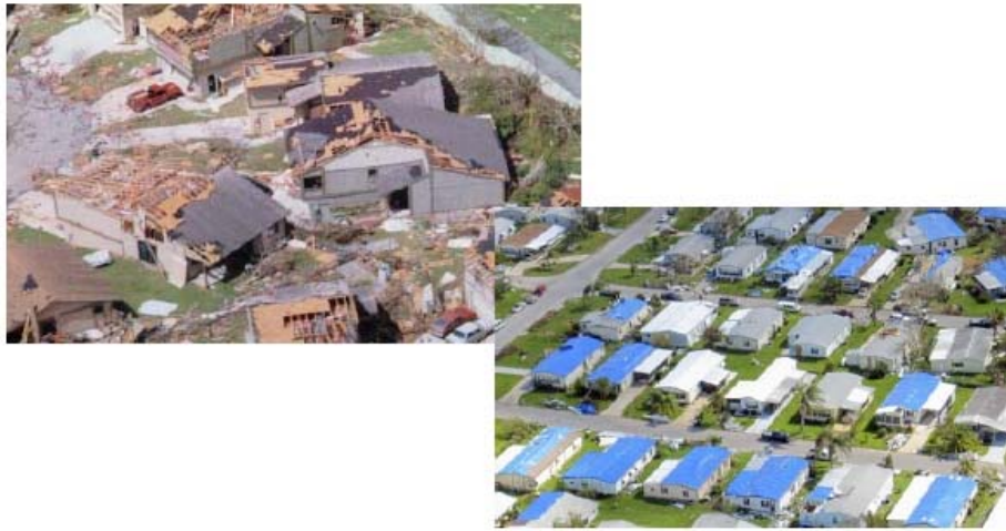
Houses with damaged or missing roof sheathing in Florida
