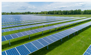
MN POWER - WRENSHALL SOLAR Wrenshall, MN Operational - 1 MWac
