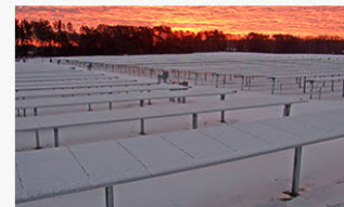
USS GOOD SOLAR Stacy, MN Operational - 1 MWac
