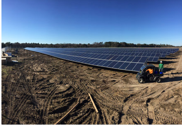
EXAMPLE OF A SOLAR PROJECT IN CONSTRUCTION
