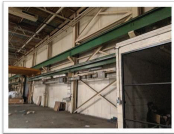
Photo #4 Existing braced frames
