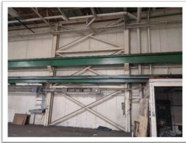
Photo #3 Existing braced frames
