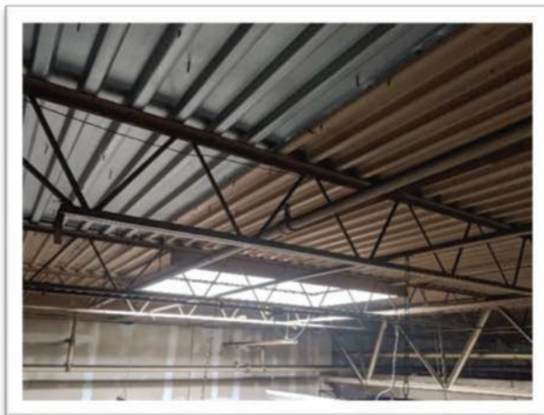
Photo #7 Existing 16-inch deep joists
