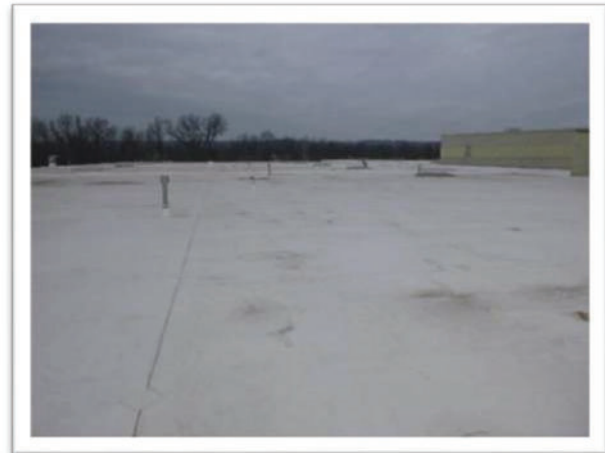
Photo #2 Flat roof proposed for solar PV
