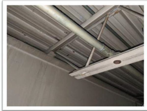
Photo #6 16-inch deep joists supported by girders
