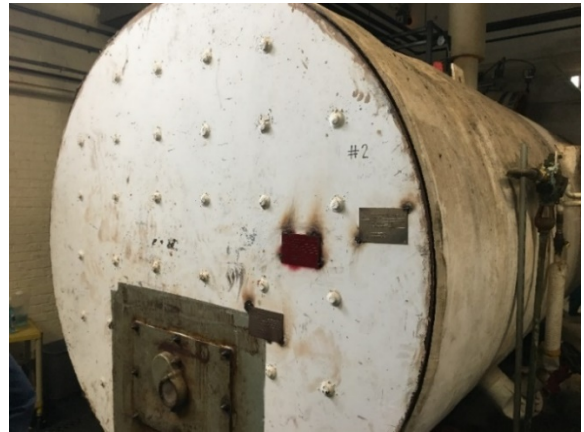
Figure 12. Franklin Steam Boiler
