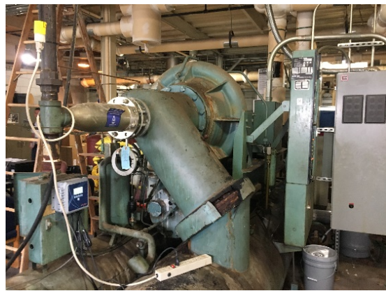
Figure 11. Cooling Tower (top) and Chiller (bottom) at Hannah Caldwell are overdue for replacement
