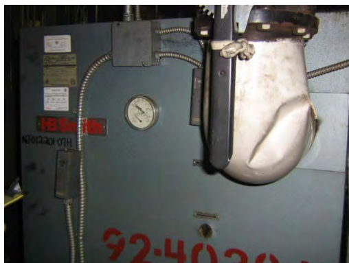
C/D wing boiler
