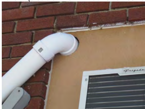
PVC pipe entering building should be sealed with foam or caulk
