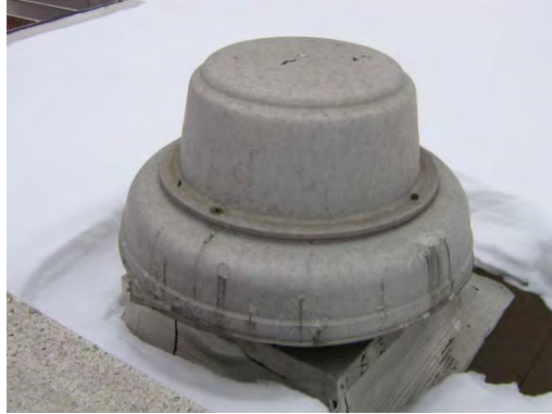
Typical Rooftop Exhaust Fan
