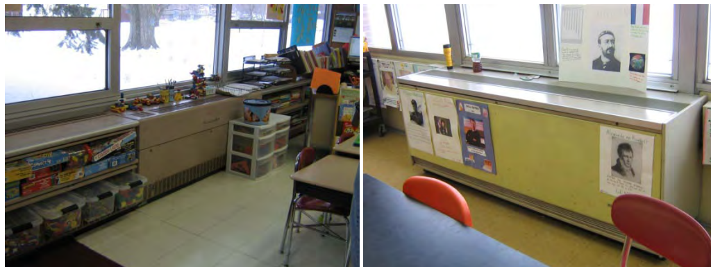
Unit Ventilators in B Wing (Left) and C Wing (Right)
