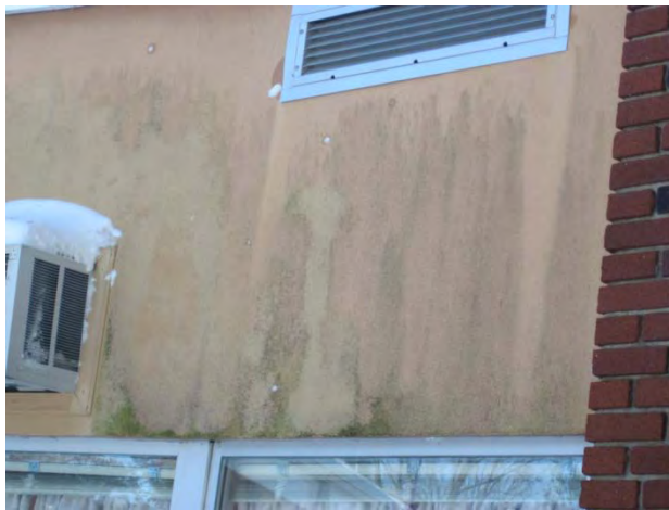
Water damage EIFS
