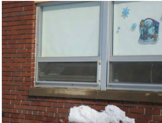
Open window on day of audit, approximately 28°F
