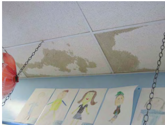
Image showing damaged ceiling tiles in classroom
