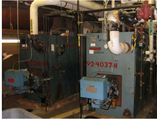
A/B wing boilers
