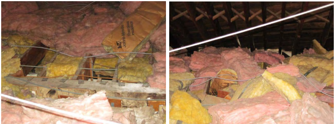
Fiberglass insulation haphazardly displaced
