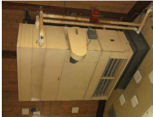
H&V Unit Suspended From Roof in Small Gym
