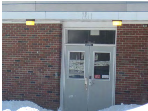
Exterior lights left on during daylight hours
