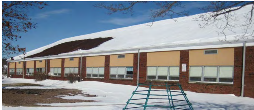
Exterior wall assembly (portion of Elementary School)
