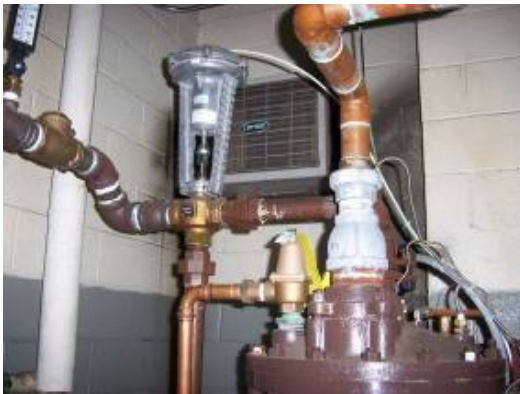
Existing Domestic Hot Water Heater
