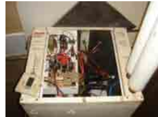
Picture: Tillis Hall Heat Pump
