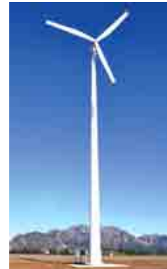
FINAL - Energy Audit Report, May 2010
