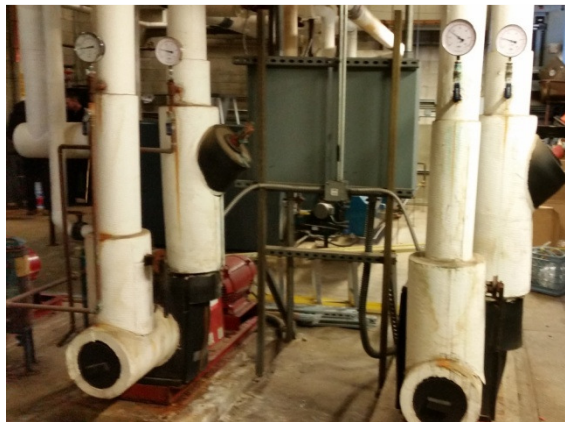
Figure M3: Existing 20HP chilled water pumps
