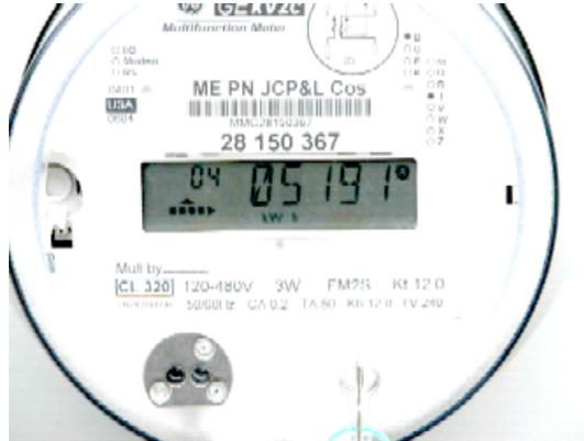
The register index in this case is the “05191”. The index is like the odometer in a car. It increases in increments only until it reaches “99999” and then it returns to zero.
