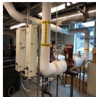
Hot Water Pumps and VFDs
