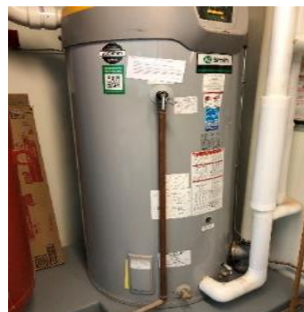
Storage Tank Water Heater
