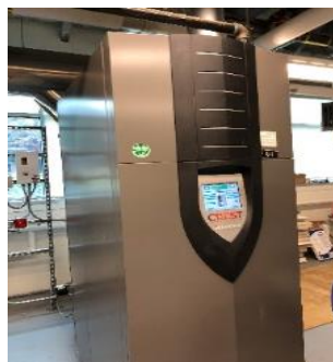
Condensing Hot Water Boiler
