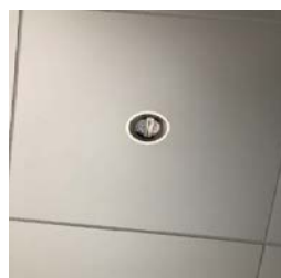
Exterior Recessed Can Fixture
