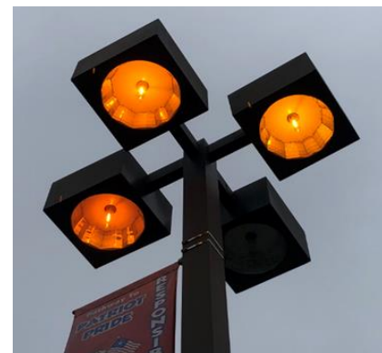
Pole Mounted HPS Lamps
