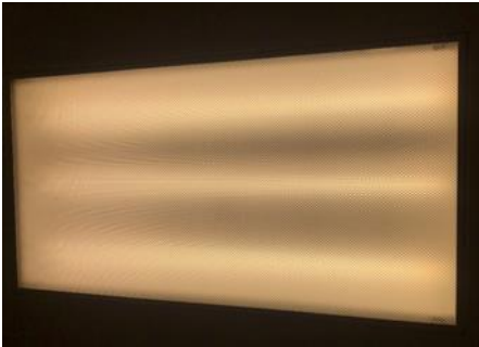
Linear T8 Troffer Fixture
