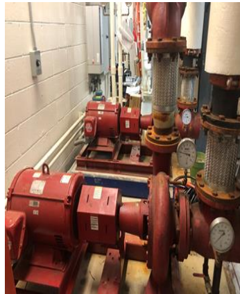
Variable Speed Water Pumps
