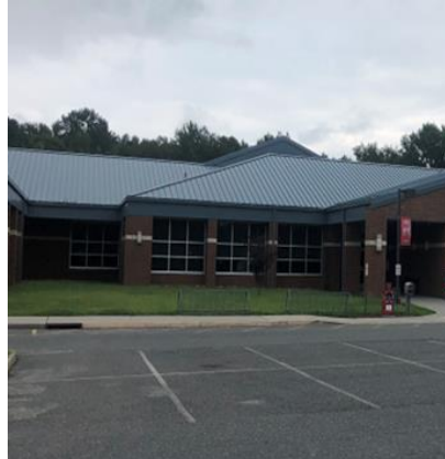
Pitched Roof with Aluminum Frames
