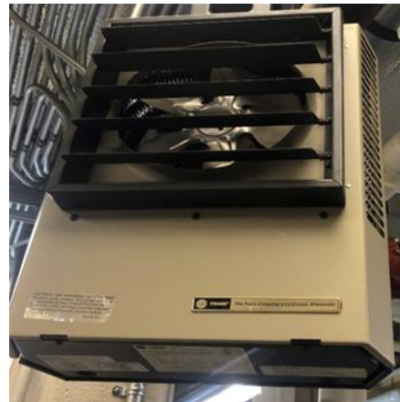
Electric Resistance Heater
