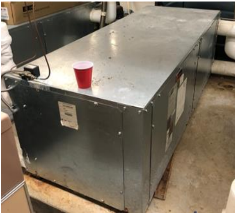
Water to Water Heat Pump
