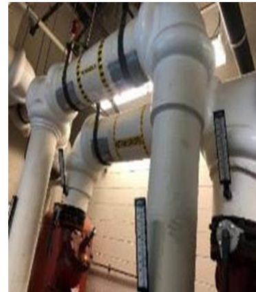
Water Source Heat Pumps Loops
