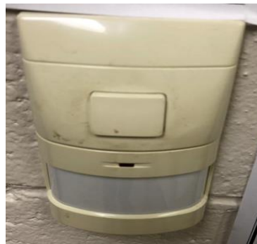
Wall Mounted Occupancy Sensor
