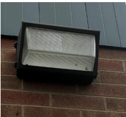
Wall Mounted LED Fixture
