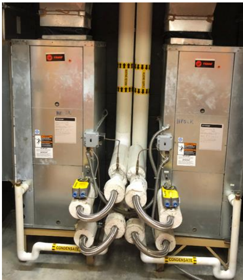
Trane Water Source Heat Pumps
