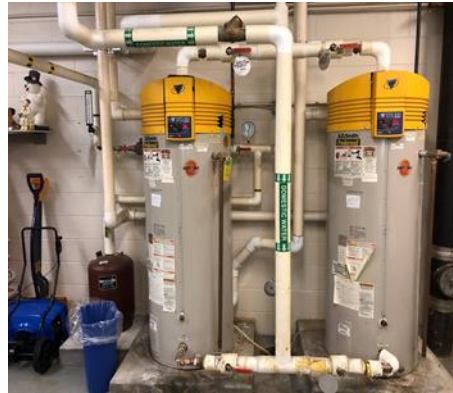
High Efficiency Domestic Water Heater
