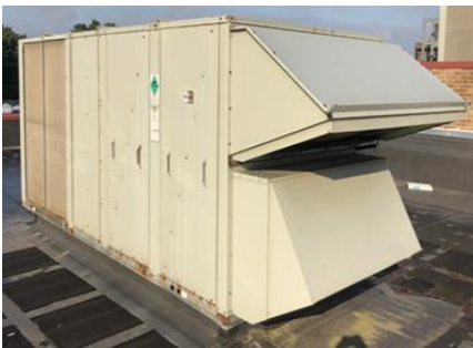
RTU with Electric Resistance Heater
