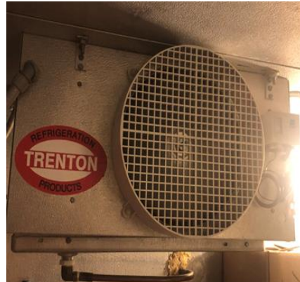
Walk-in Unit Evaporator
