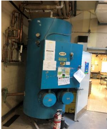
Electric Water Heater
