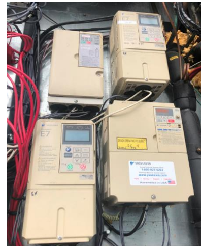
AAOV RTU with Supply & Return Fans Variable Speed Drives
