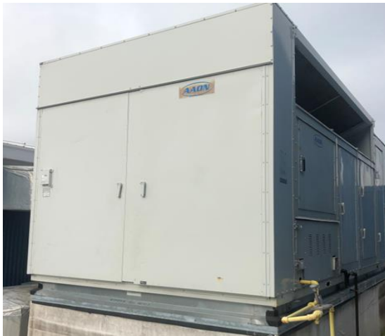
AAOV RTU with Supply & Return Fans Variable Speed Drives
