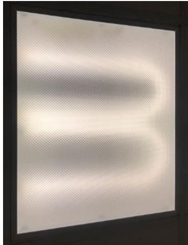
T8 with U-Shape Tubes
