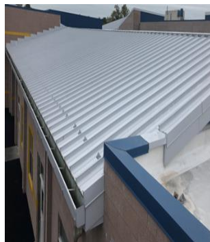
Metal Cladding Pitched Roof
