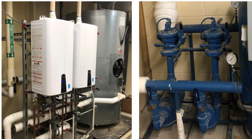
Condensing Tankless Water Heaters & Distribution Pumps
