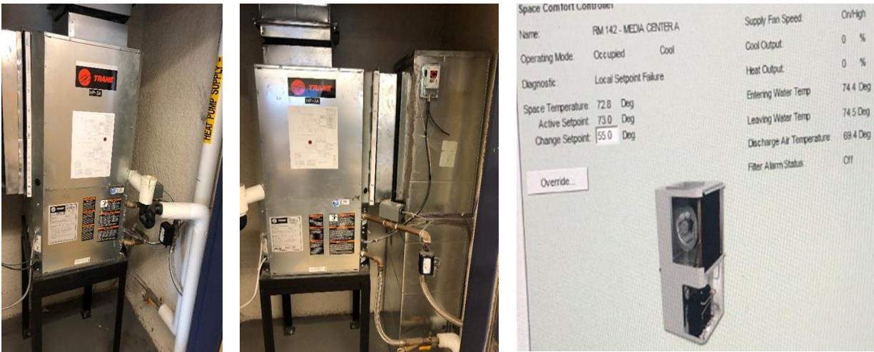
Water Source Heat Pumps & Trane EMS Control System
